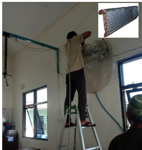
Figure 3. Evaporator cleaning process.
